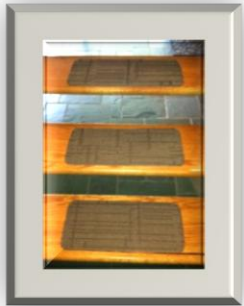
18 Staircase between floors
